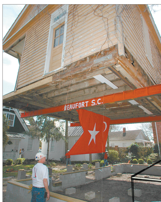
The Thomas Edmund Rhett law office was nestled into its new niche Wednesday morning by workmen with All Crane from Charleston.
